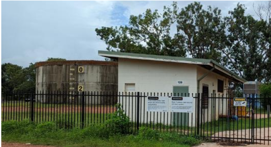
Figure 22: NASC water reservoir, pump shed and chlorination plant
