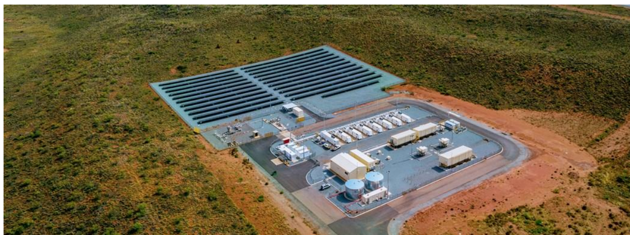
Figure 50 Onslow power station 128
