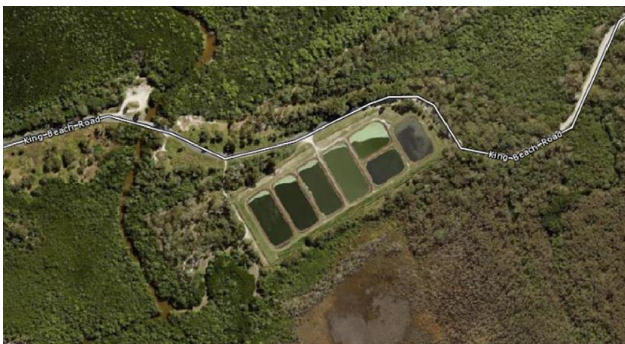
Figure 38 Yarrabah Sewerage Treatment Ponds
